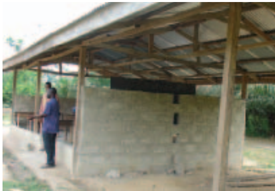
ICI has helped build six classroom blocks
